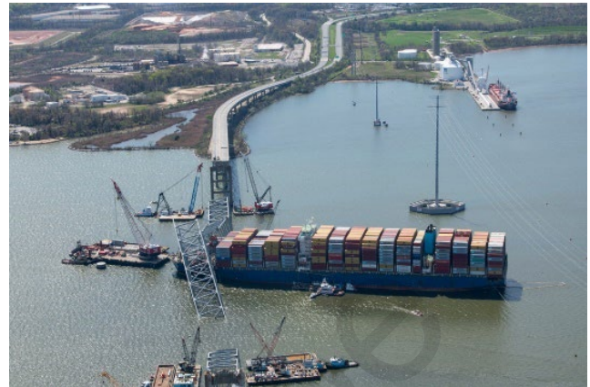
Francis Scott Key Bridge after being struck by the 'Dali' container ship, March 2024.
