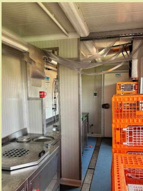
Picture 5 – Unused slaughterhouse
